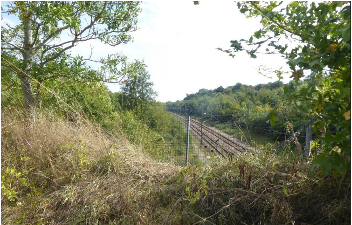
HS1 cutting from Scotland Lane land bridge, looking east – Lower Thames Crossing works would project into this cutting, providing space for Darnley Lodge Lane. Bank would be surcharged and supported by a retaining wall in the cutting.
